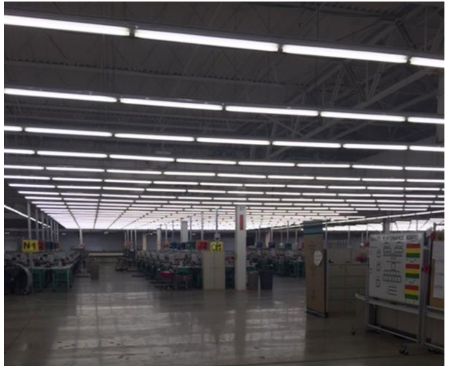
New T8 Fixtures & Ballasts Installed
