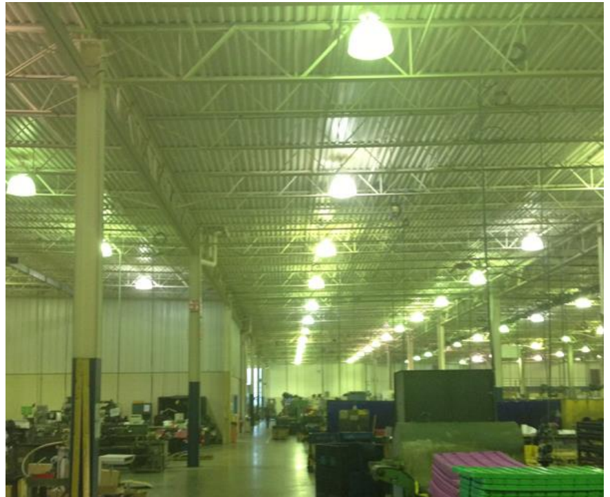
Before New Fixtures Installed
